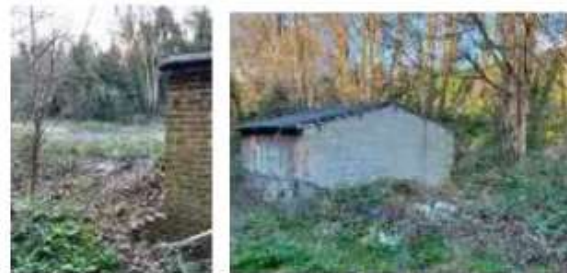
Existing brick building with bat roost potential
